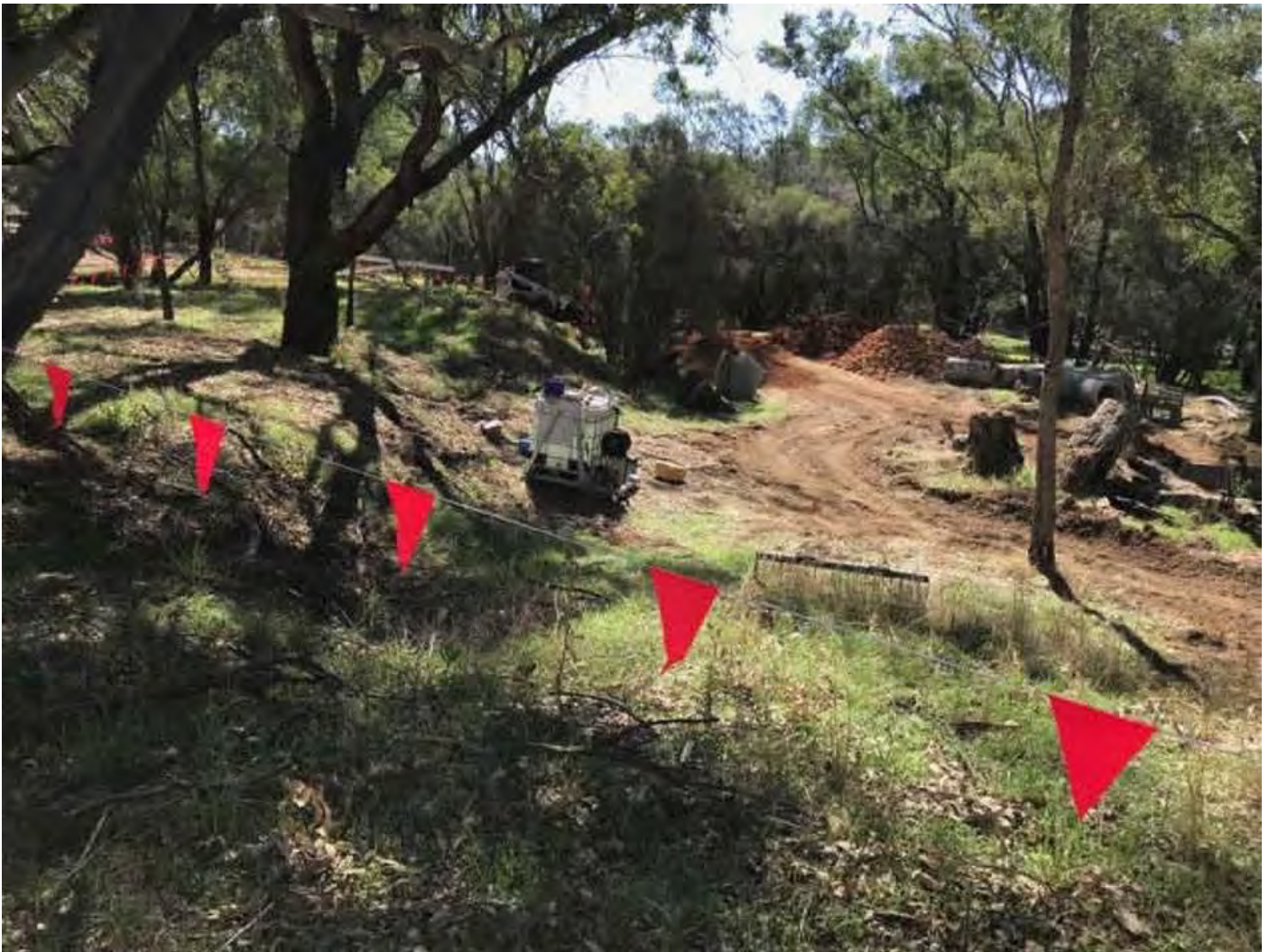
Above: The work area below the Anglican Church cordoned off.
