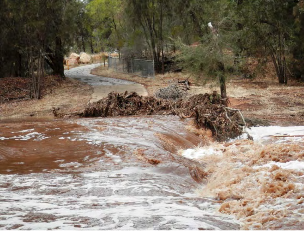
Left: Boyagerring Brook floods over the Murray Walkway during early March.
